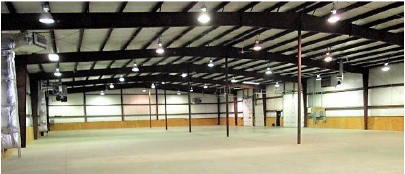
Building is 100' x 200' with 18' eave height, 2 docks and 1 drive-in door. 120/240v, 800 amp 3-phase power is available on the site.
